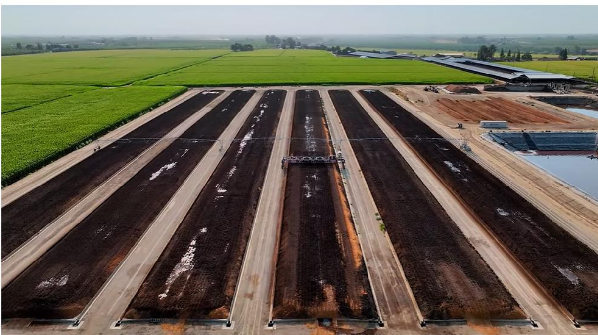
Alberto Dairy has been utilizing a BioFiltro system of six worm beds since October 2024.
